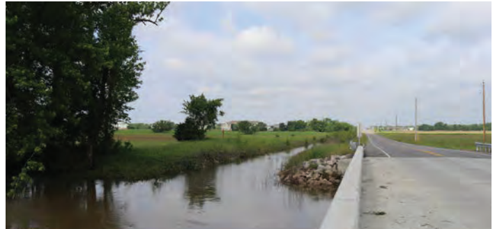
Bridge east of Ascension Via Christi Hospital
